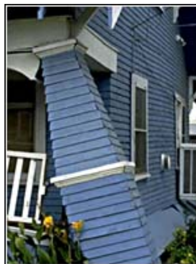
Figure 10 Earthquake Damaged Porch
